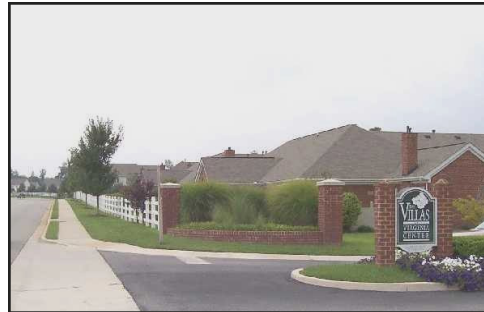
Fencing provides Access Control . The sidewalk, landscaping and sign show Territorial Reinforcement .
