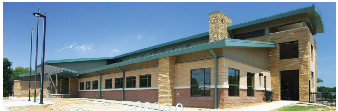
The energy-efficient Eastern Henrico Recreation Center will feature a regulation high school gym, dance studio, walking trails, football complex and other amenities.
